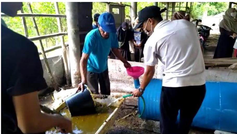
Gambar 3. Pengisian kotoran kedalam digester biogas
